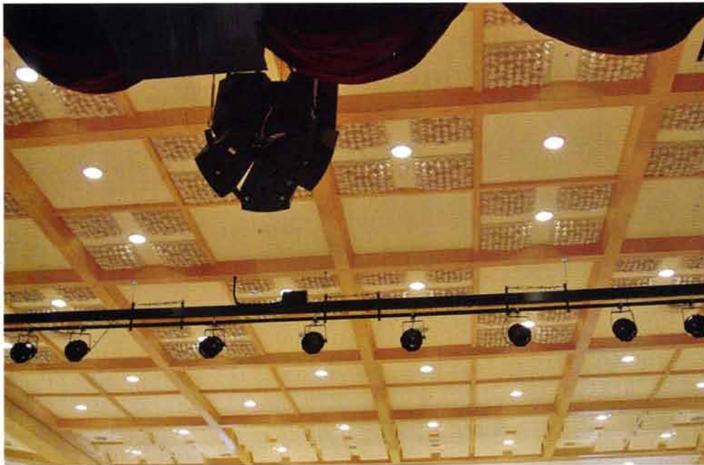
Acoustics First Model C Art Diffuser on ceiling.
