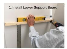
Install the wood that the Trim will "stand" on. Make sure you install it level and use the studs or drywall anchors for mounting. Countersink screws to provide a flat surface for the facing strip.
