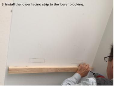
Lower facing strip should be at least 1/2" wider than the block and mounted to lower block. Make sure the 1/2" overlap is on the top. This will create a channel to hold the trim.
