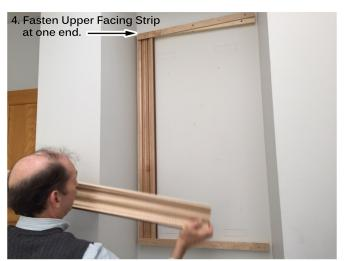
The lower facing strip should also be at least 1/2" wider than the blocking, but the overlap will be at the bottom. Attach the facing strip at one end to allow you to lift it out of the way to install the Trim.
