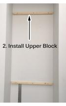
Install the wood block at the top. Make sure it is level and use the same mounting method as the lower blocking.
