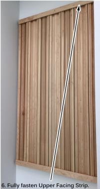
After the pieces are installed and spaced, fasten the other end of the top facing strip to hold the trim. Side blocking may be required for your install.
